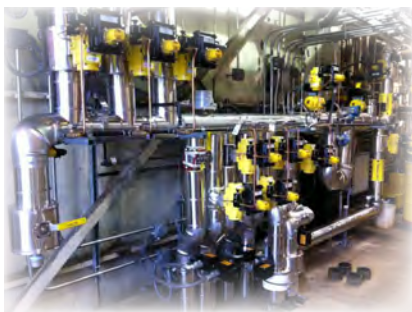
New Piping for Mesitol & Phenol System
